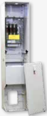
house connection pillar with HAK
