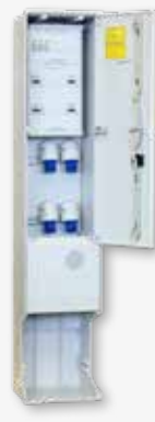
campsite distribution cabinet
