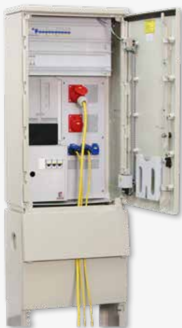
marketplace distributor with internal sockets cables are routed through the fairground base
